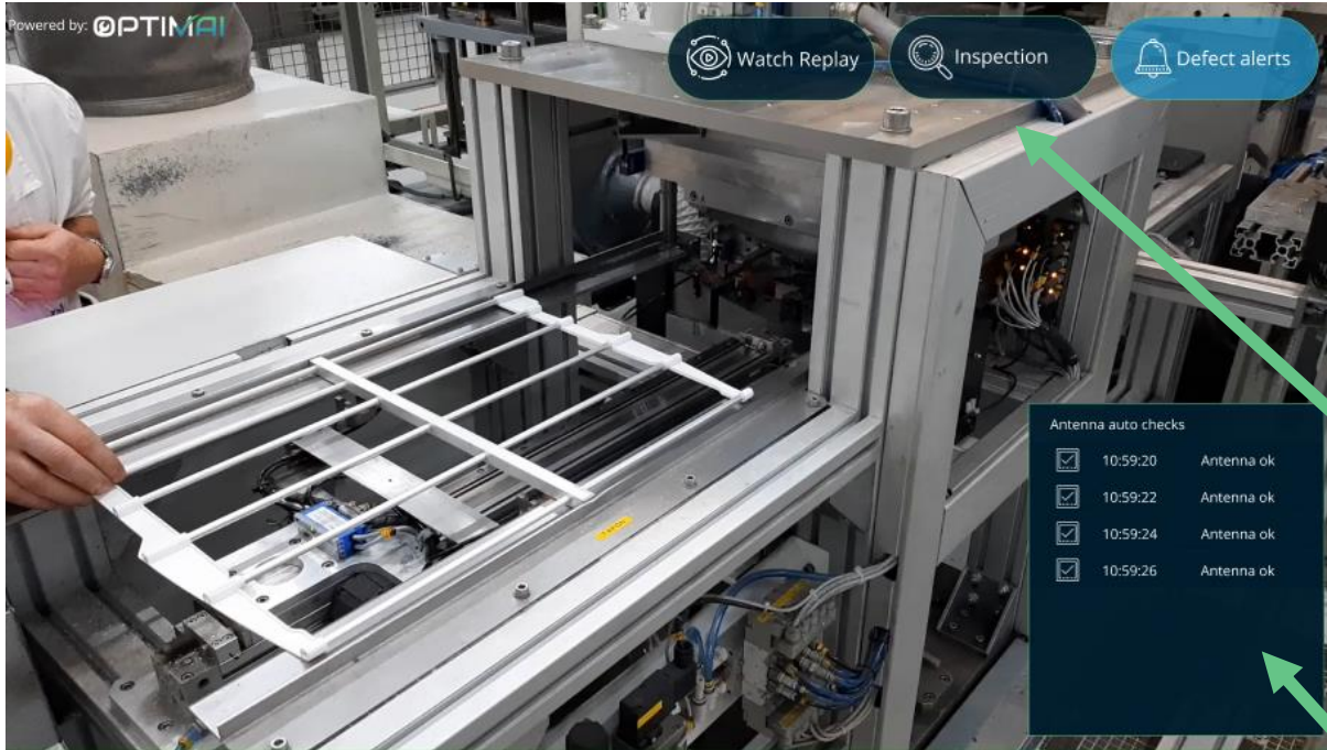
^ Antennas production line UI after the user has selected Defect Alerts tab
